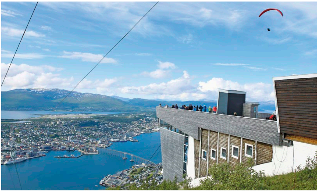
Cable car station, Tromsø
