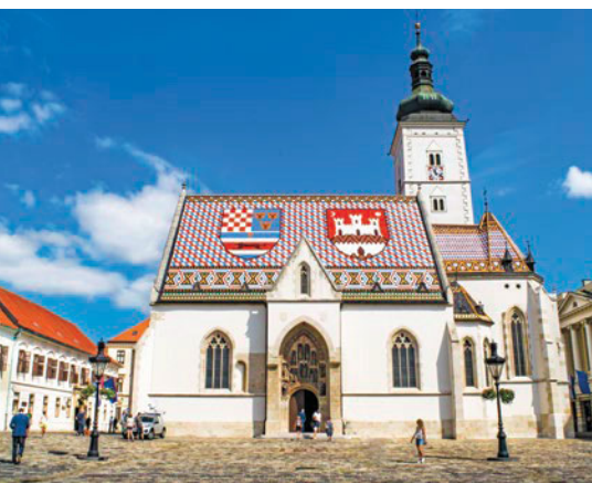
St. Mark's Church, Zagreb
